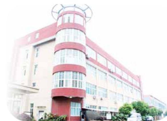
Joident's production base located at China Science and Technology Park
